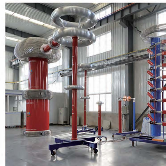
陡波冲击电压实验设备 Steep front impulse voltage test equipment
